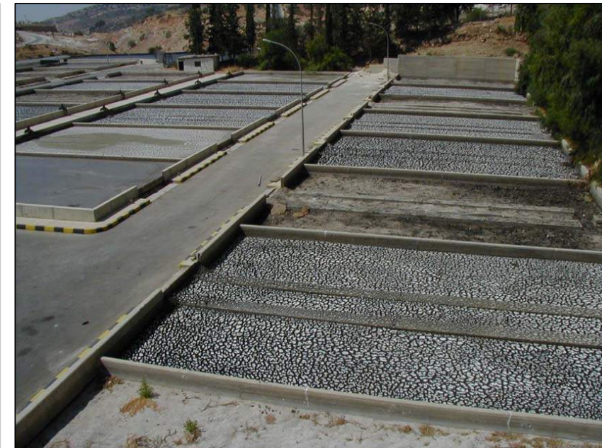
Faecal sludge drying beds - The Wadi el-Shueib Waste Water Treatment Facility- Jordan
